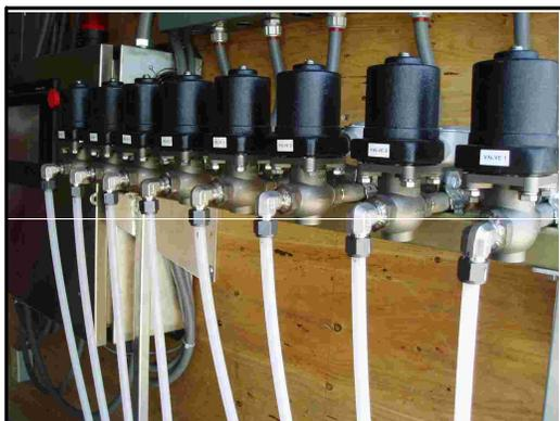
The system includes automated solenoid valves that allow pulses of concentrated ozone gas to be injected into eight sparge wells.
