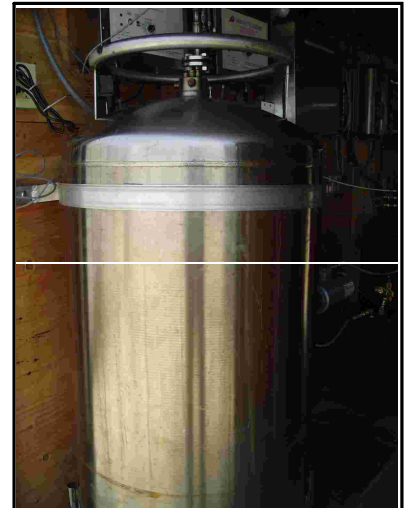
The ozone pulse-tank allows delivery of a large volume of concentrated ozone into the subsurface.
